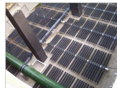
▶ 超微細気泡散気装置 (FlexAir™ MiniPanel)
